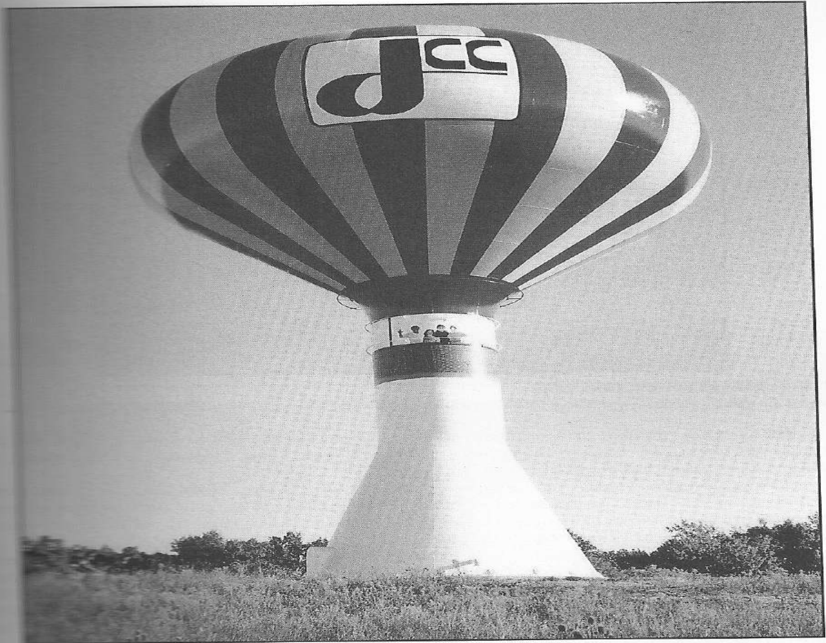
FIGURE 3-3 A 1,000,000-gal single-pedestal spheroidal elevated tank painted to look like a hot air balloon. Courtesy of CB&I
